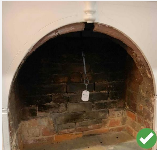
Figure 10: Fireplace without seal suitable for activity 15G
