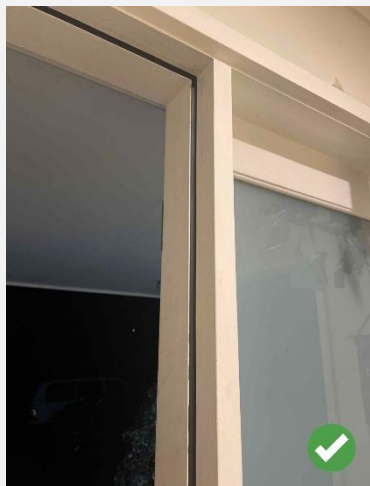
Figure 4: Post-installation photo showing weather seals on two sides of door frame (additional photo required to show whole of door frame is sealed)
