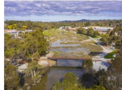
Tarralla Creek - after improvements
