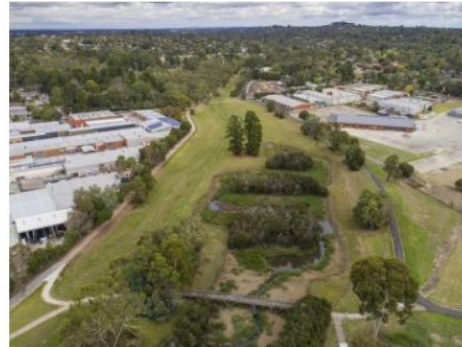
Tarralla Creek - before improvements
