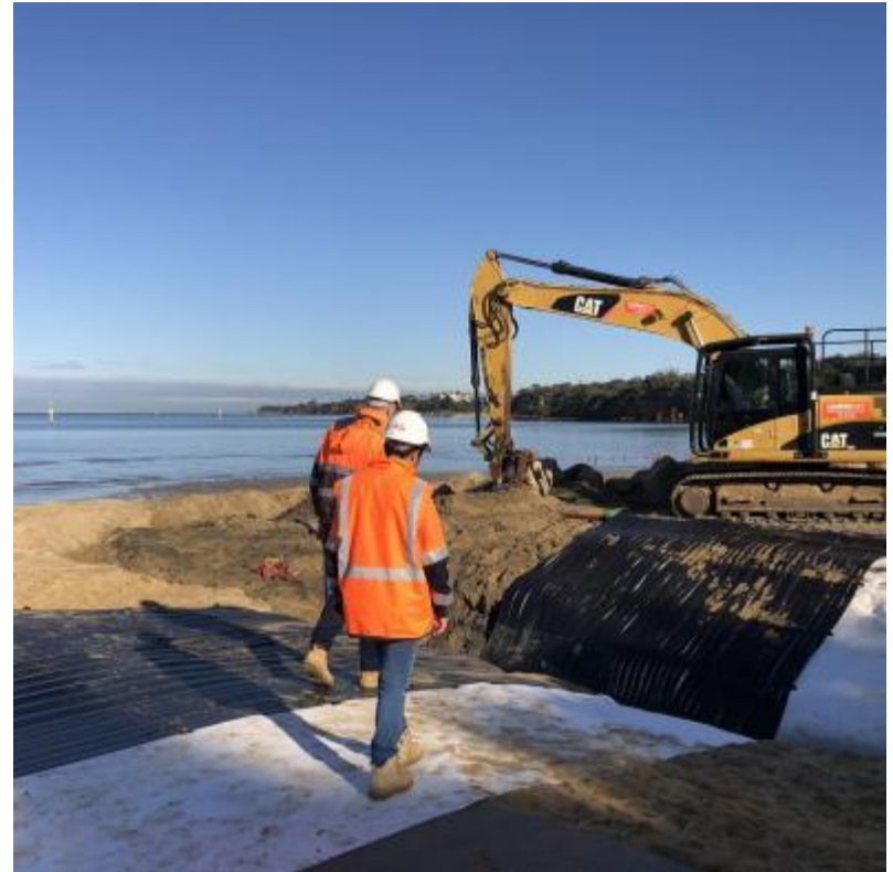
Mentone Outlet Drain Upgrade
